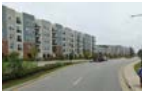
Adjacent new multifamily residential units
